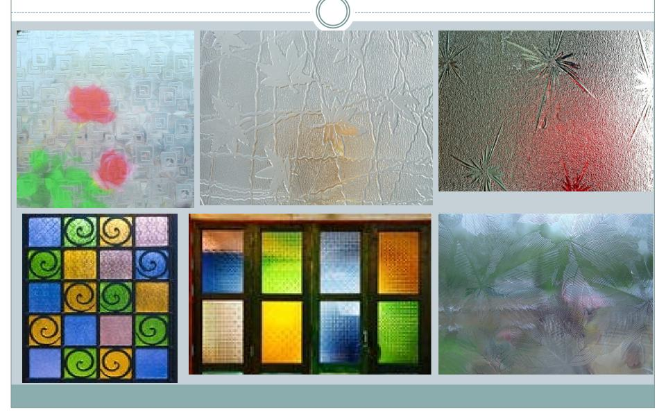
Patterned Glass is also known as Rolled or Obscure glass. It obscures a view without noticeable loss of natural or artificial light. In addition to obstructing the visibility from outside and diffusing the light, the figures soften the interior lighting. The glass achieves soft and comfortable interior lighting because its figures diffuse the incoming light. Transmission factors for solar radiation energy and visible light rays are much the same as in float glass.
